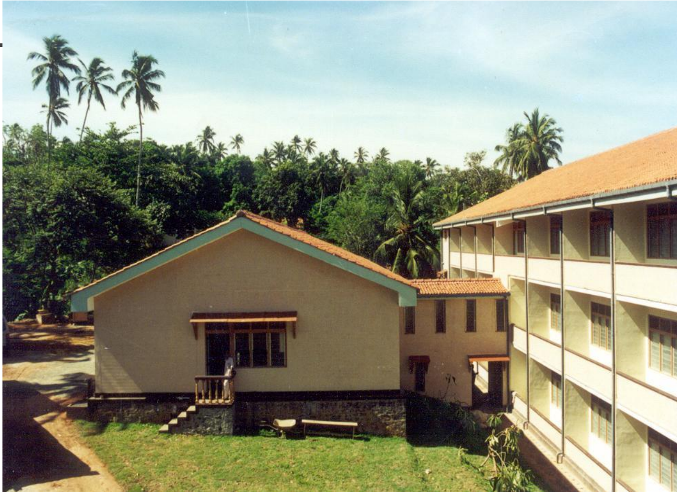
Hostel Building – University of Ruhuna
