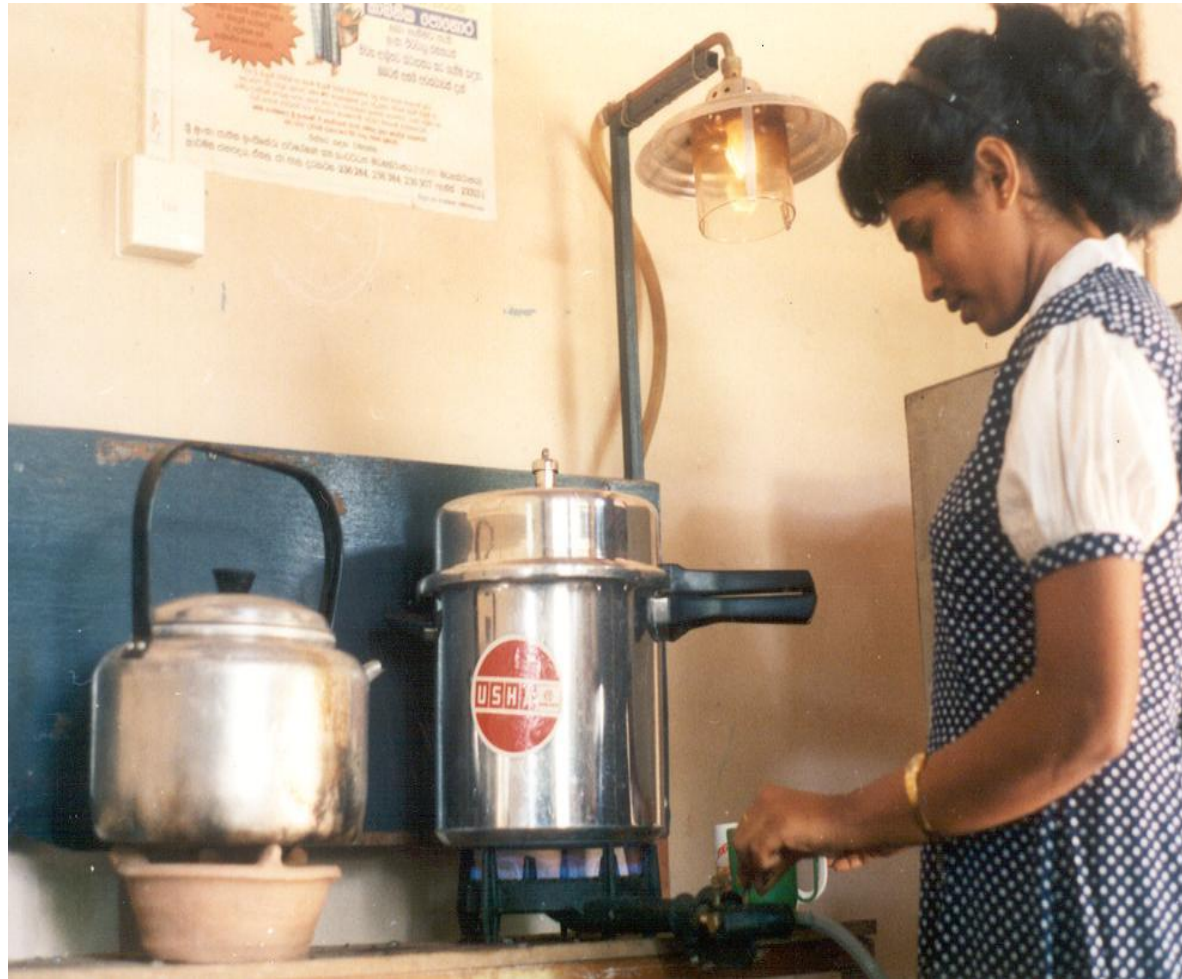
Lamp & cooker operated by using Bio gas
