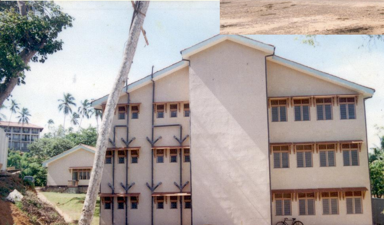
Hostel Building – University of Ruhuna
